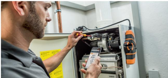
The readings are transferred wirelessly from the testo 330i via Bluetooth to the testo 330i App.
