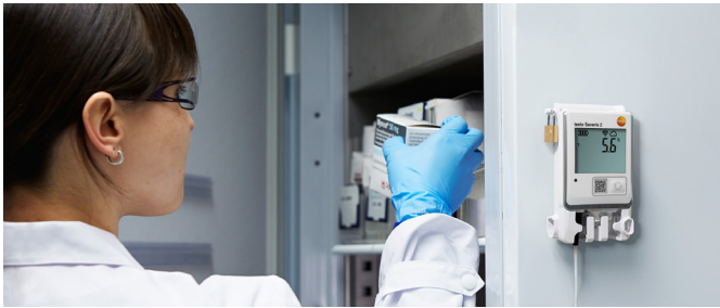
The Wi-Fi data loggers in the drugs refrigerator immediately provide the staff with an alarm when upper or lower limit values are exceeded.
