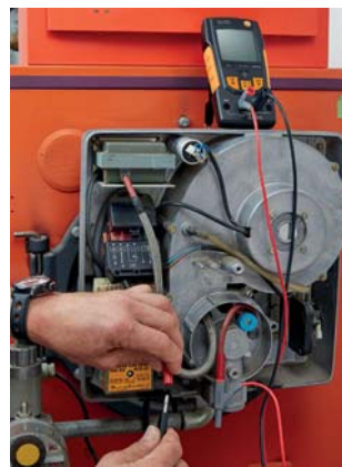
Measurement of current (µA) of burner flame rods.
