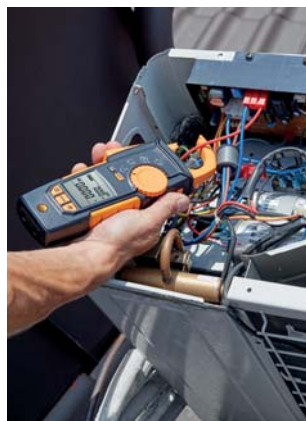
Measuring the current by clamp meter in outdoor unit of air conditioner.
