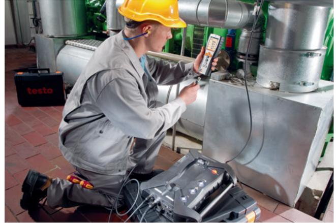
Preparation for a control measurement on a combined heat and power plant with the testo 350.
