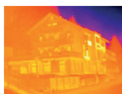
Image thermique sans testo ScaleAssist
