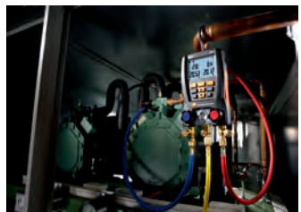
Conduct leak test
